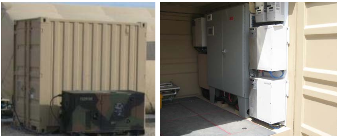
Figure 15. 10 kW hybrid system
